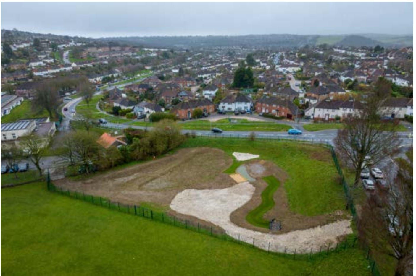
Figure 2: Site immediately after construction
